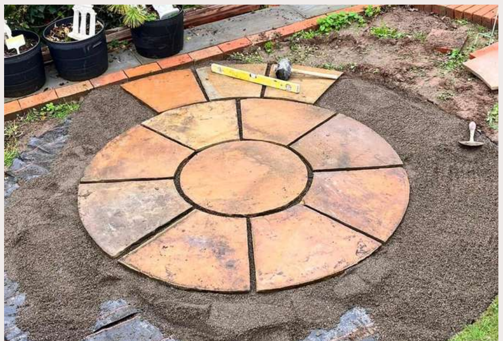
Sandstone Circle work in progress
